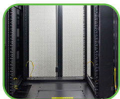
Mounting rails can be installed to allow 23" wide equipment to be installed
